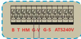
GV/GS: dry contact signal for startup the diesel generator.
